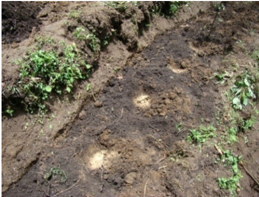
Preparation of trenches
